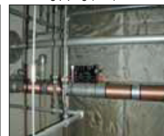
Used for the cooling towers C
